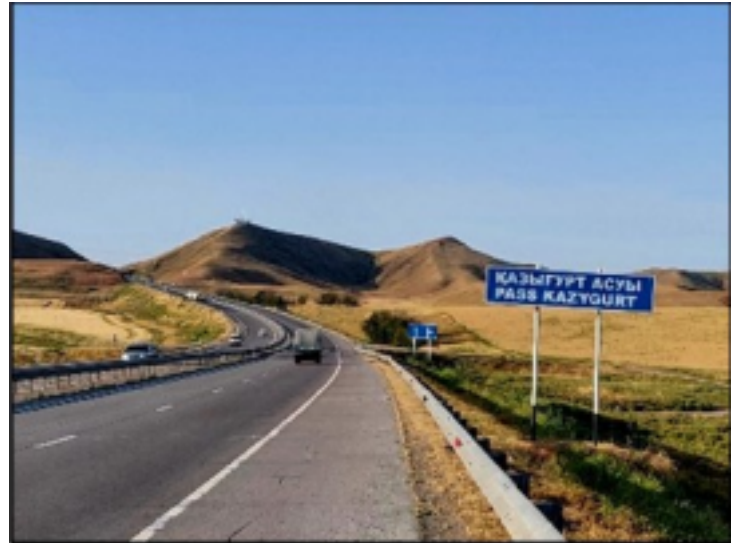
Shymkent - Tashkent Road
